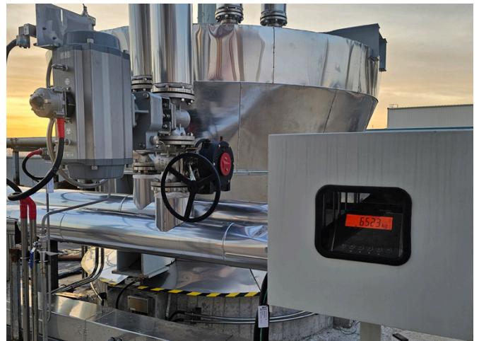
Integrated into DCS system, weighing indicators X2 enable automated control of charging and discharging process.
